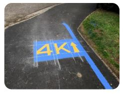
We are now working with the contractor, Wilson & Scott (Highways) Ltd, to look into more permanent painting methods (such as thermoplastic-tape and road-highway quality paints) in order to ensure longevity of the resource. On the NE route, we now have two sections painted up with an alternative paint as a test of the longevity of this solution, and are seeking funding to proceed with the re-
